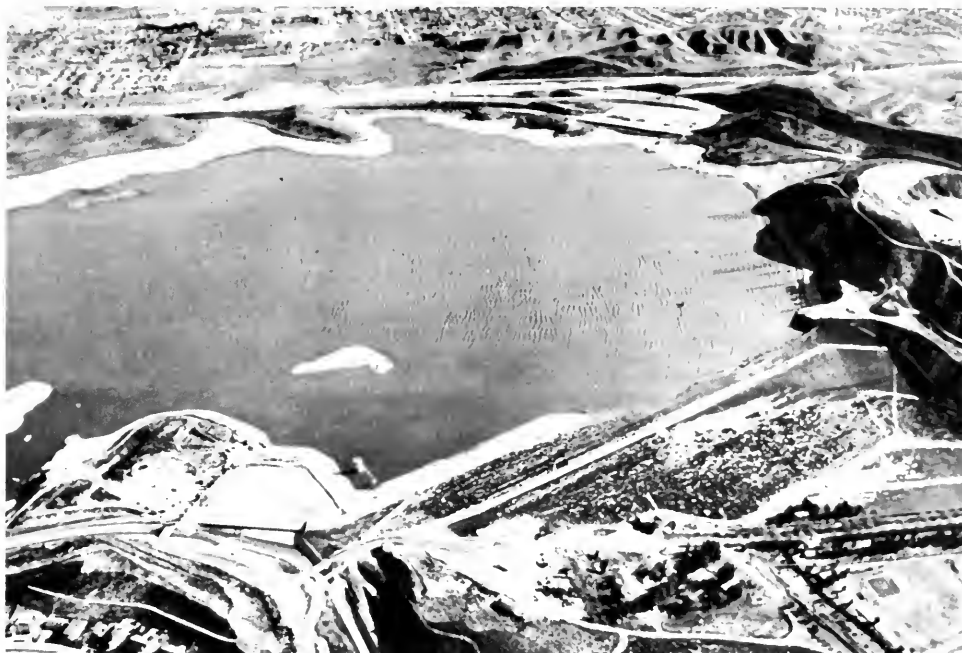
Photo 1. Aerial photo of Lower San Fernando Dam after earthquake.
